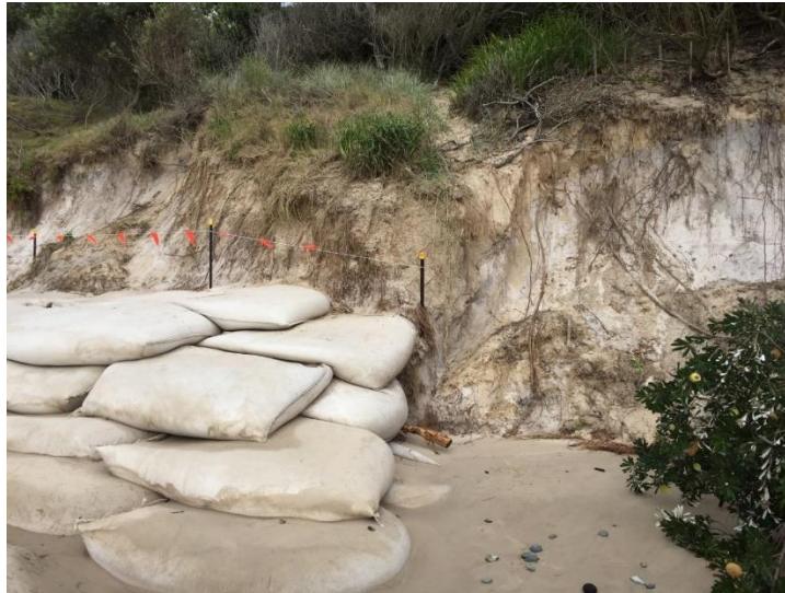
Figure 4-8 Western end of Reflections seawall (west) 2 August 2019 (within days of construction being completed)
