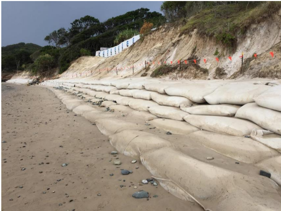
Figure 2-8 Reflections seawall (west) immediately post-construction (2 August 2019).
