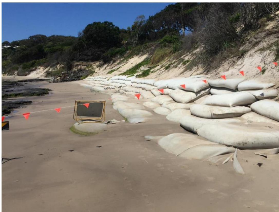
Figure 4-1 Displacement and deflation of sandbags from Reflections seawall (east) (5 November 2020)
