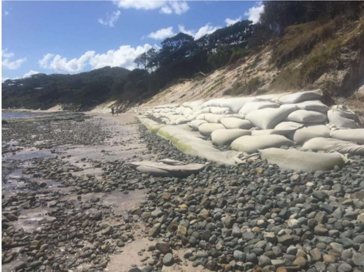
Figure 4-2 Displacement of sandbags from Reflections seawall (west) (15 October 2020)
