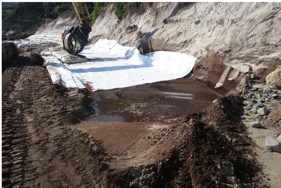
Figure 2-7 Construction of Reflections seawall (east) with geotextile filter directly overlying the clay layer. July 2019.
