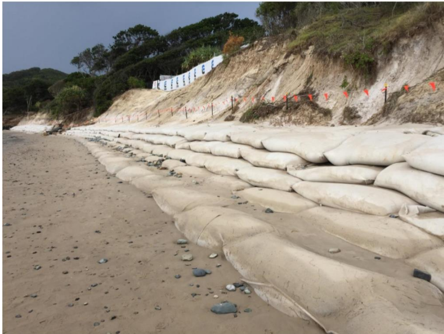
Figure 2 Reflections seawall (west) – immediately post construction (August 2019)
